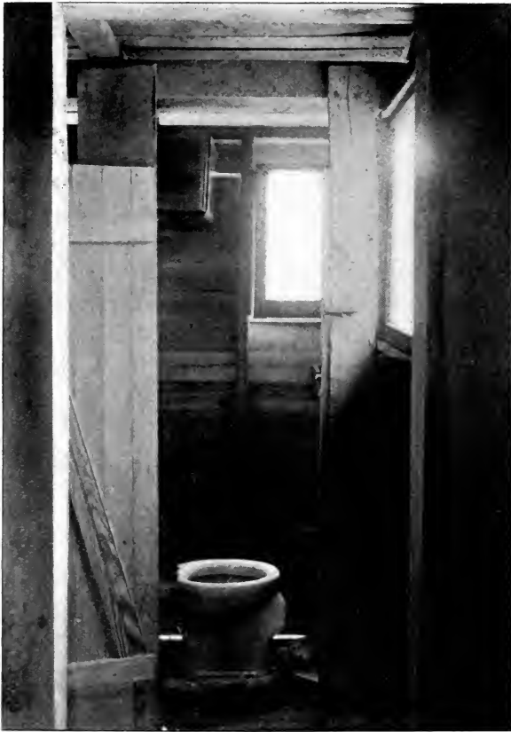
FLIMSY CONSTRUCTION OF COMPARTMENTS, AND POOR INSTALLATION OF PLUMBING. TOILET SEAT BROKEN OFF (SECOND TOILET AT LEFT). DWARF DOORS, INADEQUATE PRIVACY, AS TWO TOILETS ARE USED BY BOTH SEXES (SEE NEXT PICTURE FOR OUTSIDE CONSTRUCTION)
