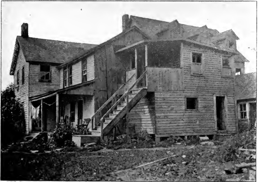
FLIMSY CONSTRUCTION OF ADDITIONS; BACK YARD GARBAGE STREWN AND SATURATED WITH SLOPS
