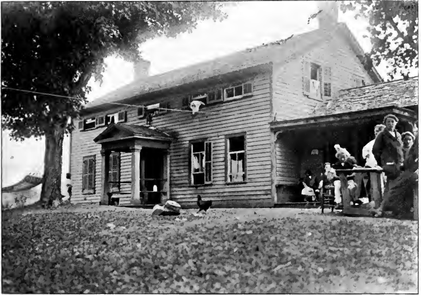
TEN BEDROOMS, ONE FAMILY IN EACH, WITH COMMON KITCHEN AND DINING ROOM; 15 TO 20 ADULTS; 30 TO 40 CHILDREN. WATER SUPPLY, A SPRING WHICH RECEIVES SURFACE DRAINAGE AND WASTE FROM KITCHEN SINK; ONE PRIVY WITH LOOSELY BUILT REMOVAL DRAWER, OVERFLOWING AT TIME OF INSPECTION
