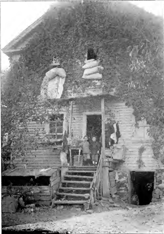
TENEMENT CONDITIONS IN A VILLAGE. BEDDING IN WINDOWS; FOOD BOX ON PORCH; GARBAGE THROWN IN YARD; 2 TO 4 TENANTS PER ROOM
