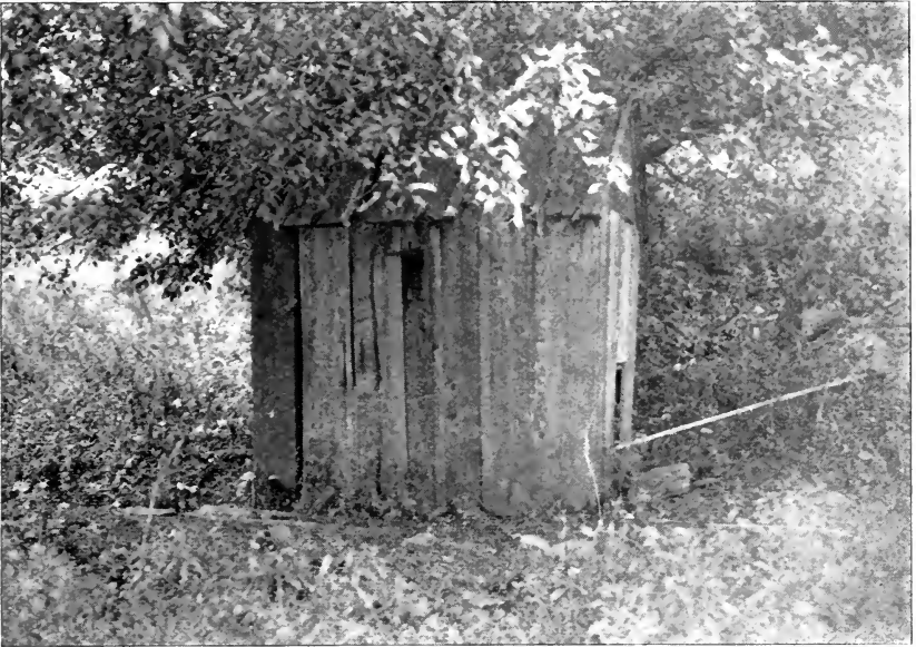
SHELTER OVER SPRING AT FOOT OF HILL. BOARDS OF SHELTER ROTTED AT BOTTOM. GROUND AROUND SPRING, DEEP MUCK. SPRING ONLY WATER SUPPLY FOR 10 FAMILIES IN HOUSE. RECEIVES SURFACE DRAINAGE FROM YARD, TWO PRIVIES AND KITCHEN SINK
