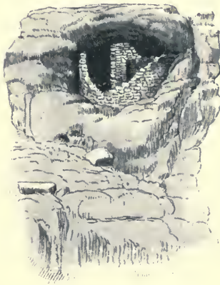
Fig. 74. Cliff-dwelling on the Rio Mancos.
