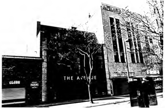
Figure 35: "The Avenue" Dress Shop (Formerly Coward Shoe Store) Oscar Stonorov and Louis I. Kahn, archts., 1949.
