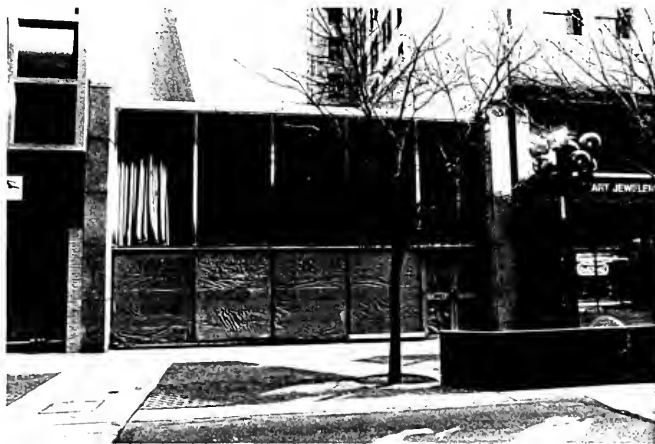
Figure 72. Mercantile Library: View of Main Elevation. [Photo taken by author.]
