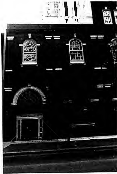
Figure 28: Addition to Provident Bank Bldg. (Built 1947) [Photo taken by author.]
