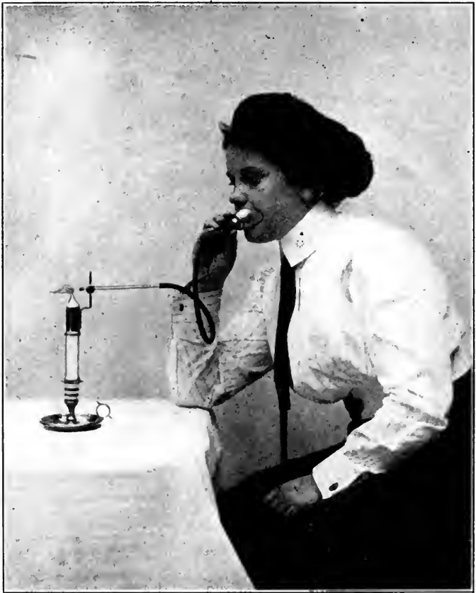
FIG. 42. — Candle flame indicator used for the mouth.
