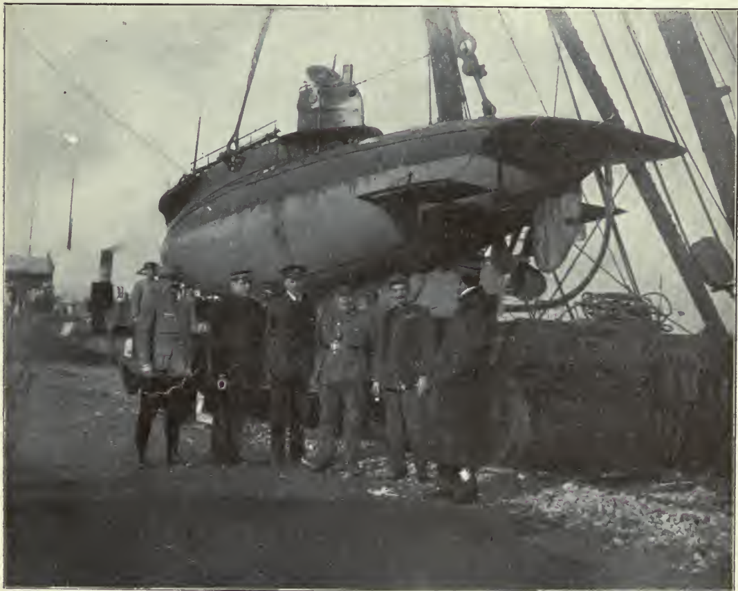
One of the small submarines being hoisted from the quay into the water.
