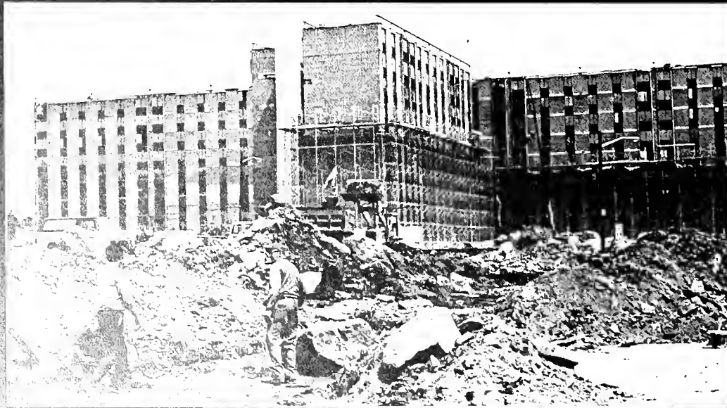
Construction of the Reservoir Apartments
