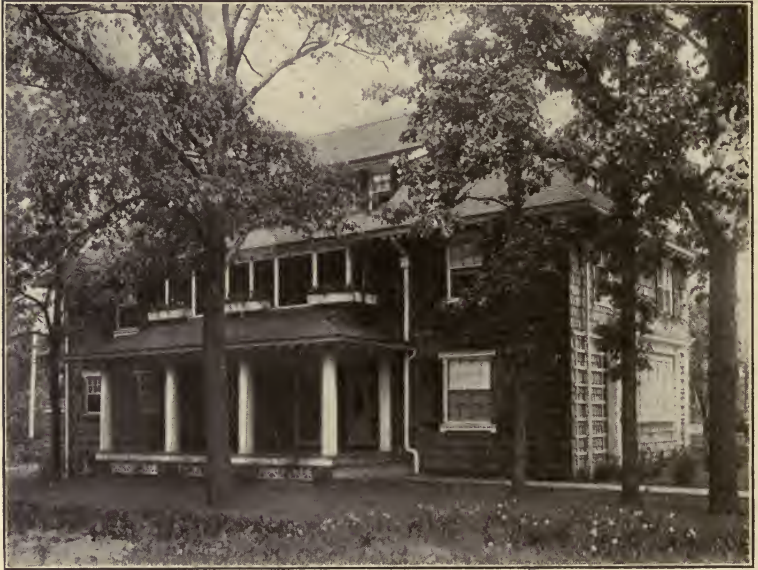
GALVANIZED IRON GUTTER AND CORNICE.
