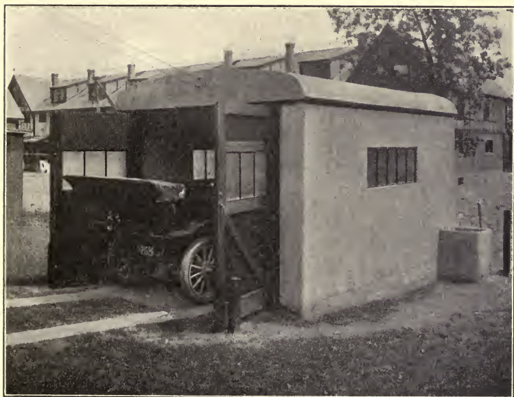
METAL FRAME PLASTERED GARAGE.
