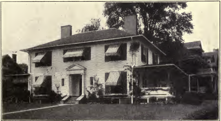
SHINGLE ROOF WITH HANGING METAL GUTTER.
