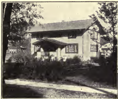
CEMENT-PLASTERED HOUSE OF MODERATE COST.
