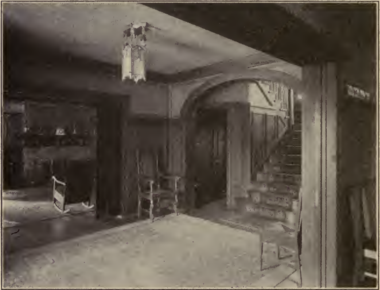
OAK WAINSCOT ON A STAIRCASE.
