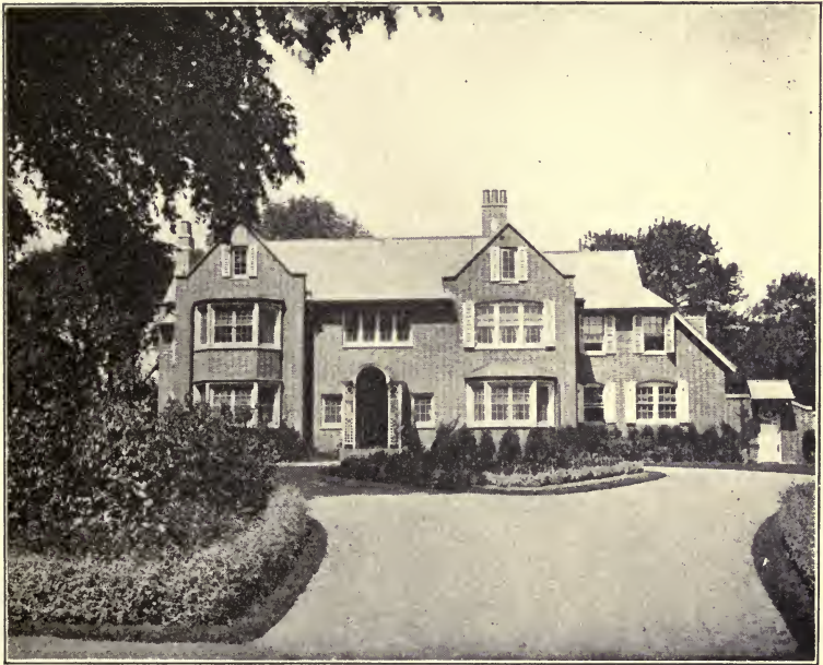
BRICK COUNTRY HOUSE NEAR BOSTON.
