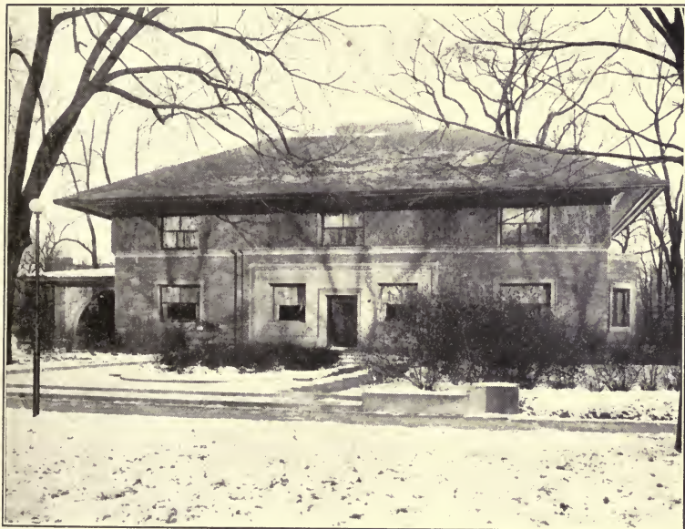
THE DIGNITY OF ROMAN BRICK WITH LIMESTONE TRIMMINGS.
