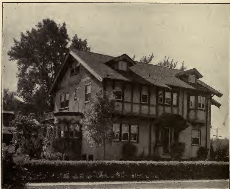
BUILT-IN GUTTERS LINED WITH COPPER.
