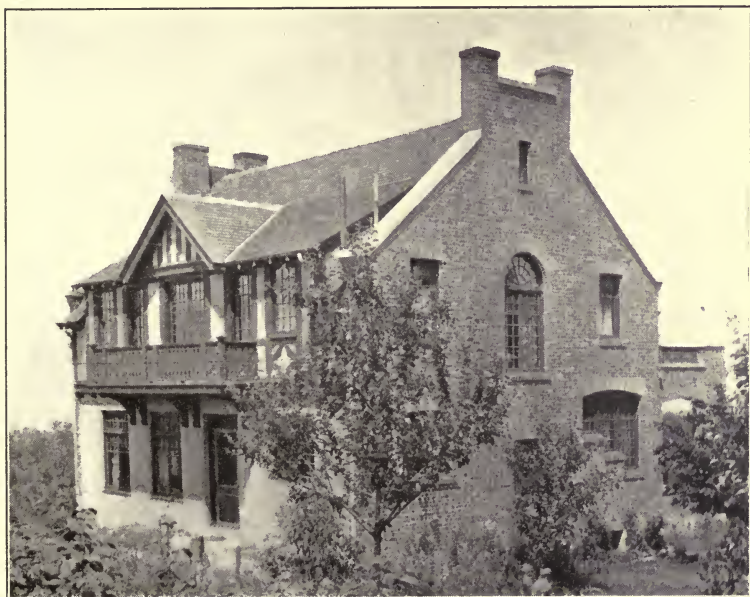
PLUMBING STACKS EXTENDING ABOVE ROOF.
