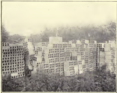
HOLLOW TILE STACKED READY FOR USE IN A FIREPROOF HOUSE.
