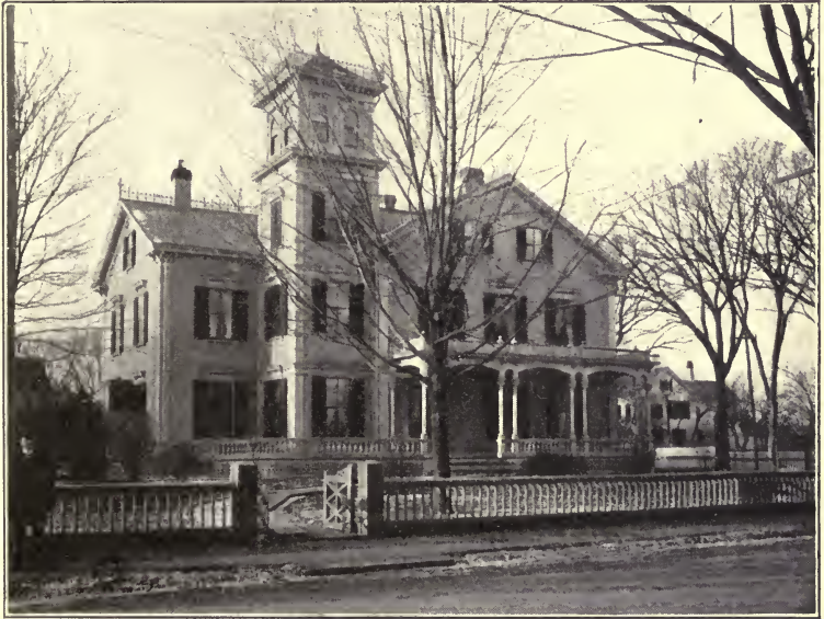
OLD HOUSE BEFORE REMODELING.
