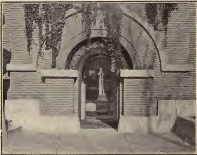
MOLDED BRICK ARCH OVER AN ENTRANCE.
