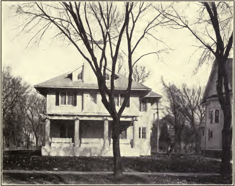
VERANDA ON END OF HOUSE.
