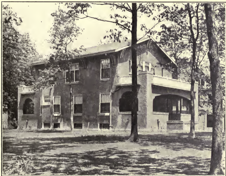
STEEL FRAME HOUSE COMPLETED.
