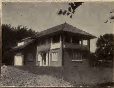
LARGE BRICK GARAGE.
