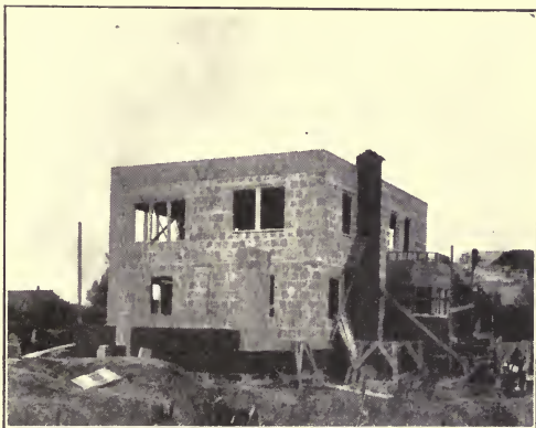
TILE HOUSE IN PROCESS OF CONSTRUCTION.
