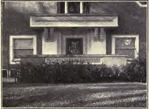
DOME LIGHT AT ENTRANCE.
