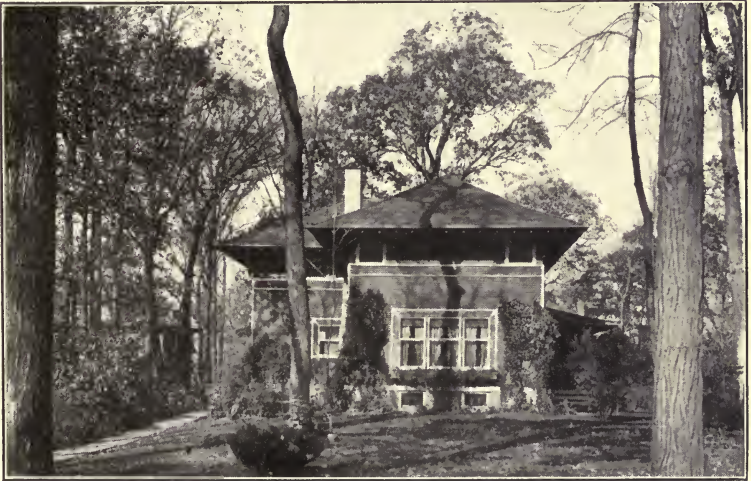
NARROW SIDING WITH CORNER BOARDS.
