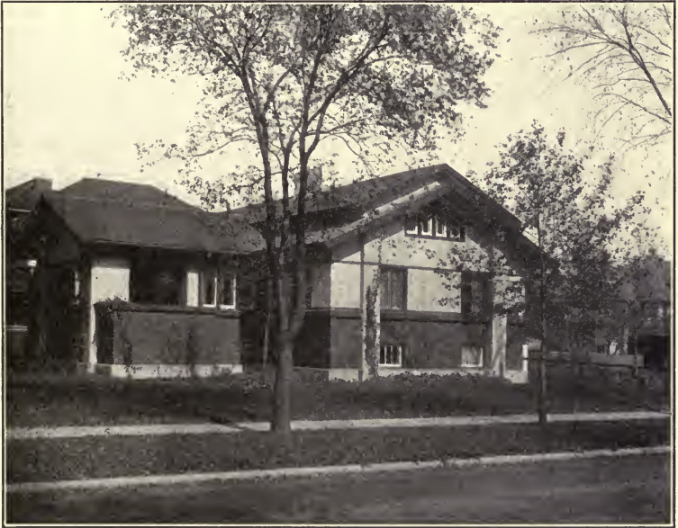
GREEN STAIN ON SHINGLES AND ROUGH-SAWED TRIM.
