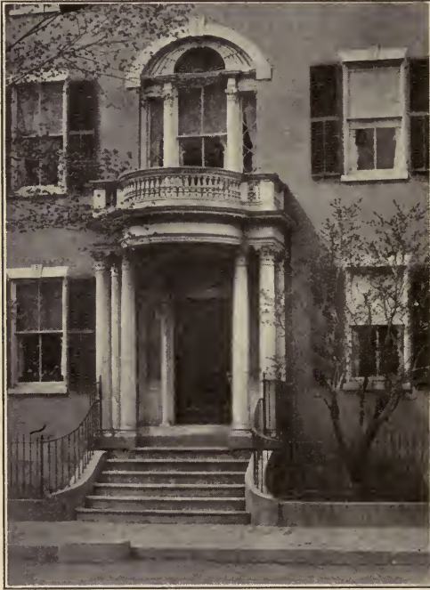
COLONIAL DOORWAY ON AN OLD SALEM HOUSE.
