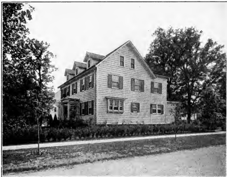
GREEN SHUTTERS ON A WHITE HOUSE.
