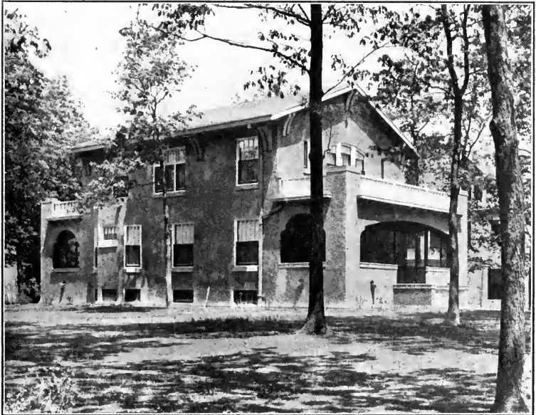
STEEL FRAME HOUSE COMPLETED.
