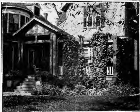
NEW PORCH ON AN OLD HOUSE.
