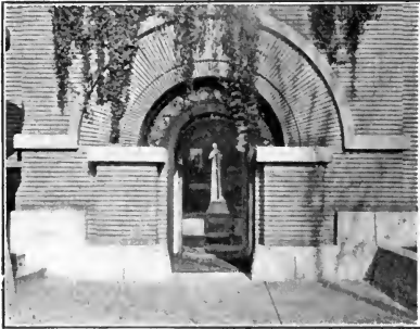
MOLDED BRICK ARCH OVER AN ENTRANCE.
