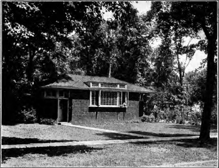
A LITTLE BUNGALOW OF SHINGLES.
