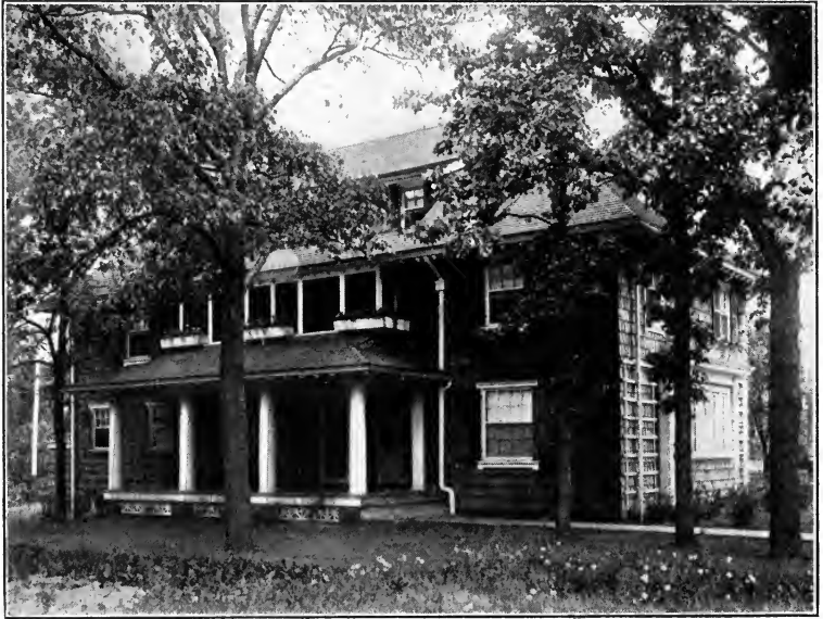
GALVANIZED IRON GUTTER AND CORNICE.
