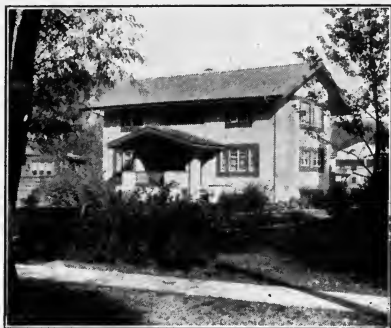
CEMENT-PLASTERED HOUSE OF MODERATE COST.
