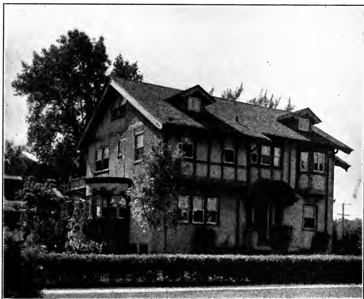
BUILT-IN GUTTERS LINED WITH COPPER.
