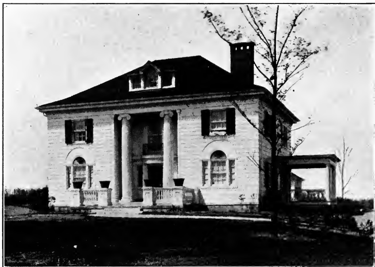
SIDING WITH MITERED CORNERS.
