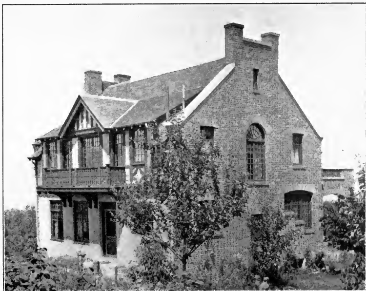
PLUMBING STACKS EXTENDING ABOVE ROOF.
