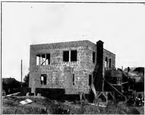
TILE HOUSE IN PROCESS OF CONSTRUCTION.
