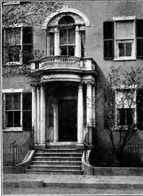
COLONIAL DOORWAY ON AN OLD SALEM HOUSE.
