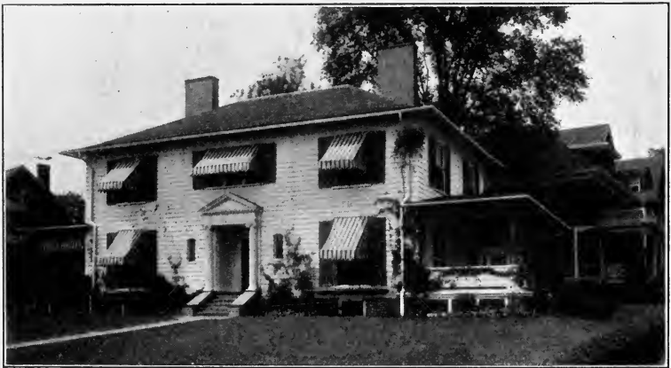
SHINGLE ROOF WITH HANGING METAL GUTTER.
