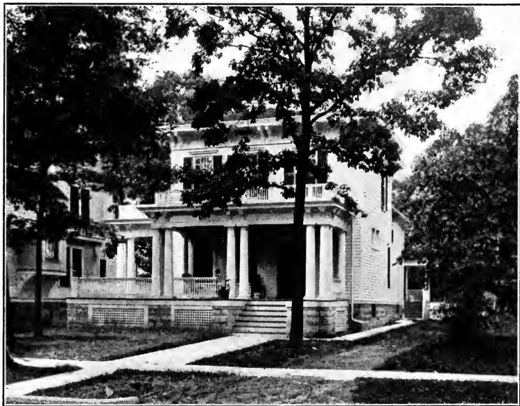
PLAIN HOUSE REMODELED.
