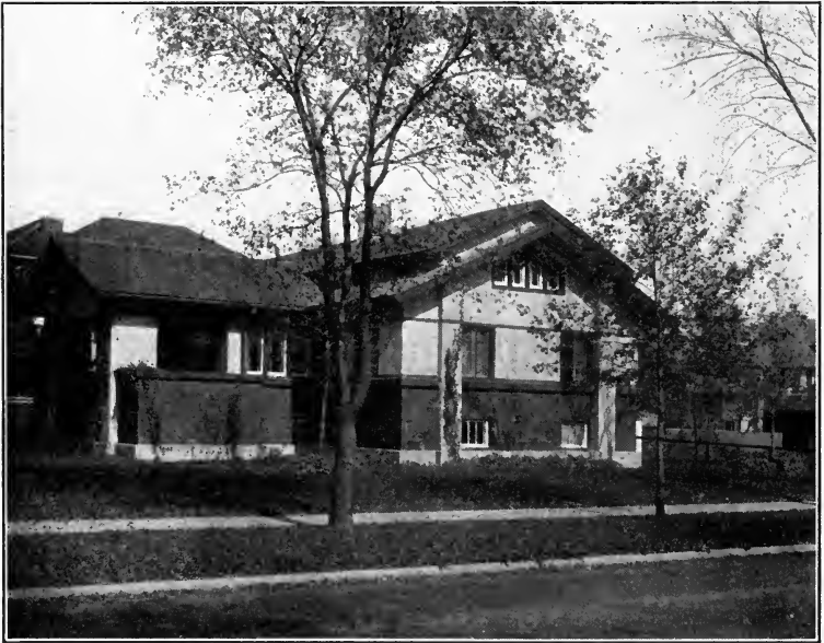
GREEN STAIN ON SHINGLES AND ROUGH-SAWED TRIM.
