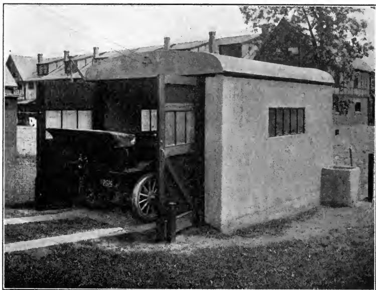
METAL FRAME PLASTERED GARAGE.
