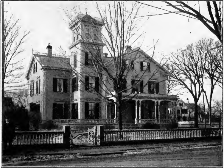
OLD HOUSE BEFORE REMODELING.
