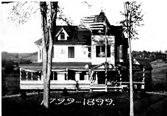
RESIDENCE OF THE LATE GENERAL WILLIAM W. GROUT, KIRBY, VERMONT.
