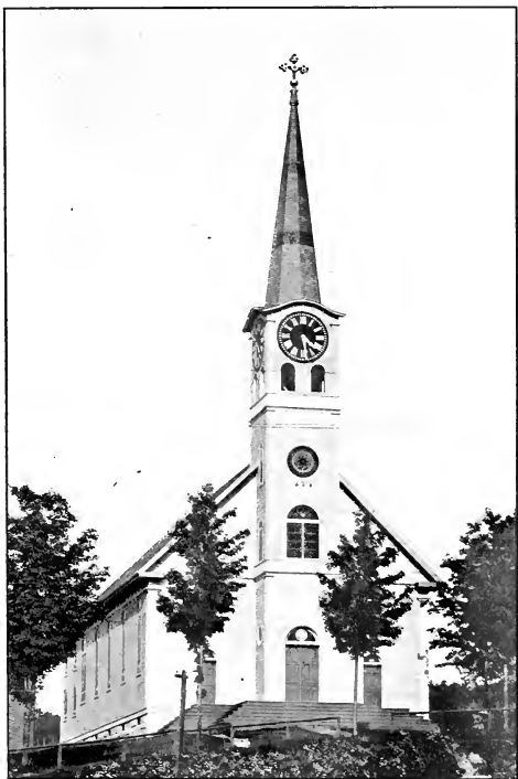
ST. PAUL'S CATHOLIC CHURCH, BARTON, VERMONT.
