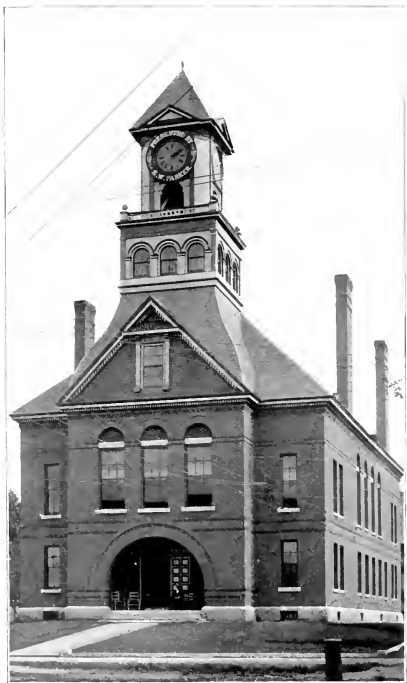
ORLEANS COUNTY COURT HOUSE, NEWPORT.
