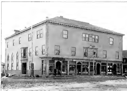
OPERA HOUSE BLOCK, ISLAND POND.
