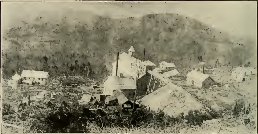
ASBESTOS MINES AT EDEN, OWNED BY BEN B. BLAKE.
