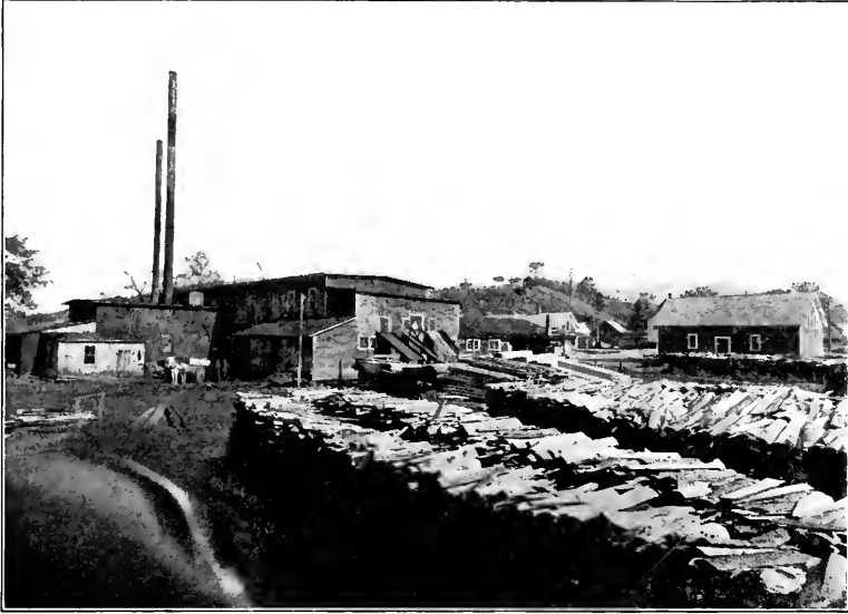
MILL OF L. BAKER & SONS, AT EAST RICHFORD.
