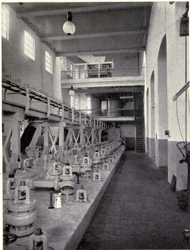
The floor above the Diffusers, in which the juice is extracted from the Beet slices.
