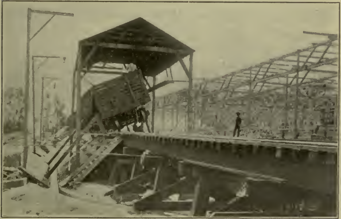
PLATE XVI. — Above , beet dump in common use in many sections, California; below , car dump with hydraulic jack, California. (Courtesy Truman G. Palmer.)
