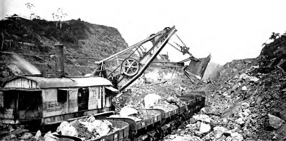
STEAM SHOVEL IN THE CULEBRA CUT.
