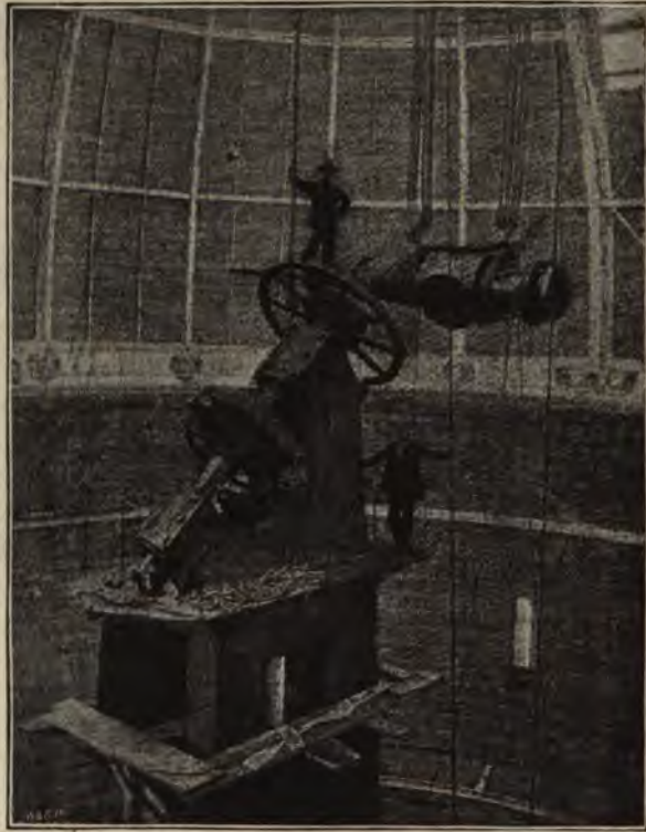
FIG. 1.—Erecting the declination axis of the Yerkes 40-inch refractor.
