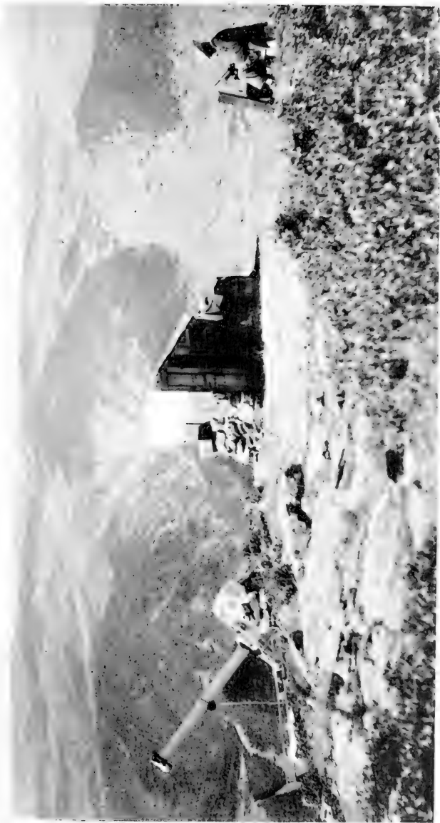
Smithsonian solar-radiation expedition to Bassour, Algeria, 1911. Prof. Brackett observing with the silver-disk pyrheliometer. The instrument shelter is weighted with stones to prevent its being blown away.
