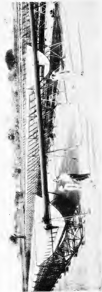
The Shuman-Boys solar engine at Meadi, Egypt, 1913. (After Ackermann. From "The Earth and the Stars," courtesy of the Van Nostrand Co.)
