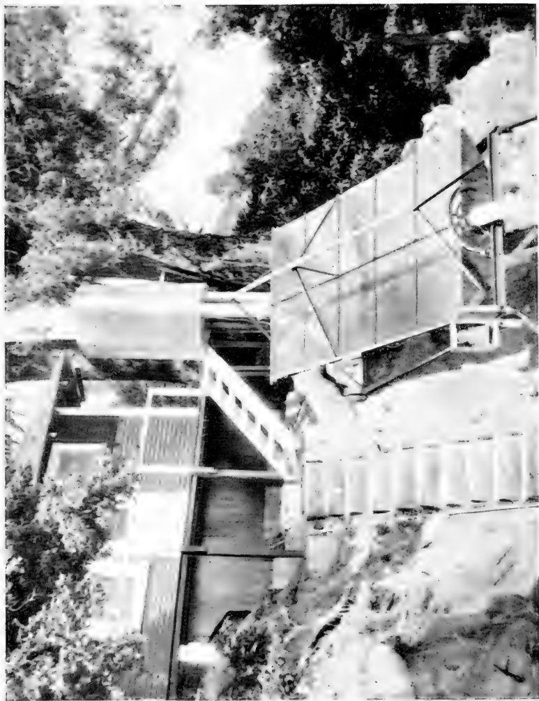
Abbot's solar cooker. Rays caught by the great mirror heat oil in the focus tube. The oil, circulating, bathes the cooking ovens in the reservoir above. The ovens stay heated night as well as day, and bake bread, meat, etc.
