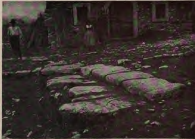
FIGURE 7.— ANCIENT ROAD-PAVEMENT AT THE THIRD FORK, 17
