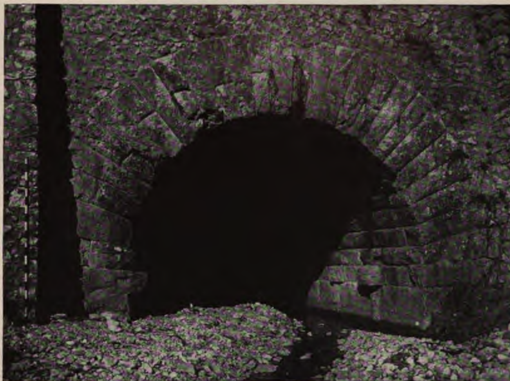
FIGURE 1. — PONTE DI SAN GIORGIO, VIEWED FROM THE EAST Only the arch of travertine is Roman
