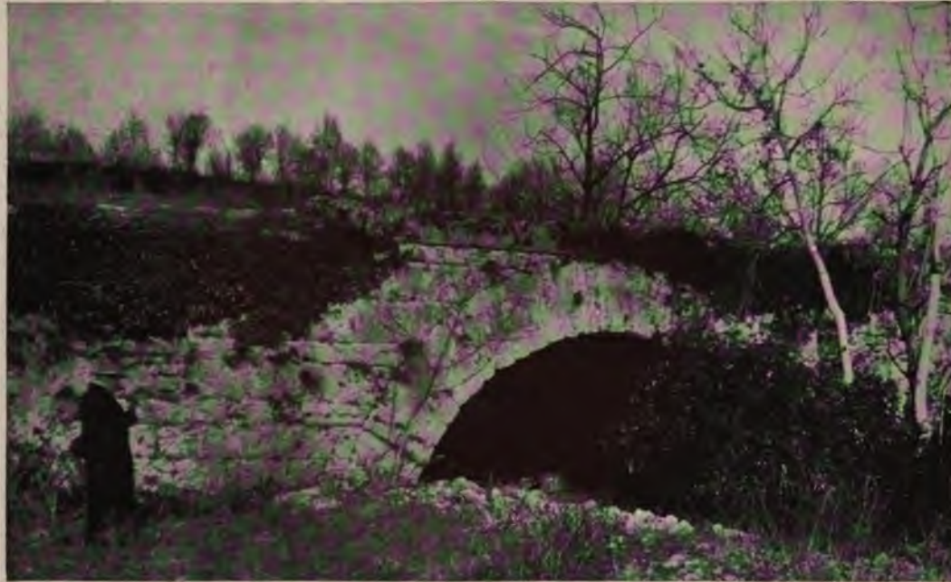
FIGURE 2.—PONTE SCUTONICO, BUILT OF TRAVERTINE, VIEWED FROM THE SOUTHEAST
