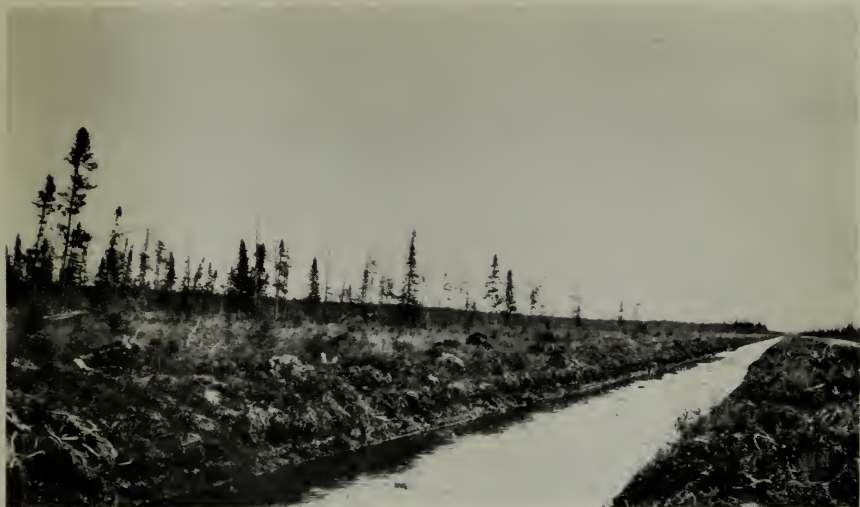
A. DRAINING A MUSKEG SWAMP IN ROSEAU COUNTY
