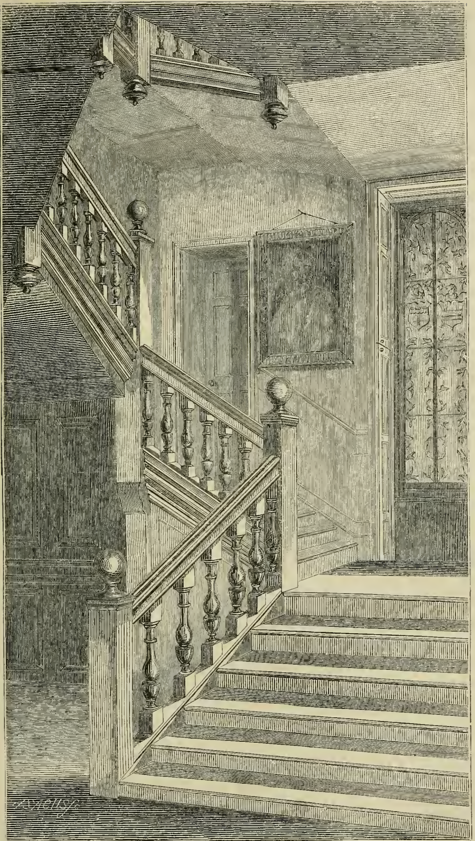
STAIRCASE IN TRADESCANT'S HOUSE.
