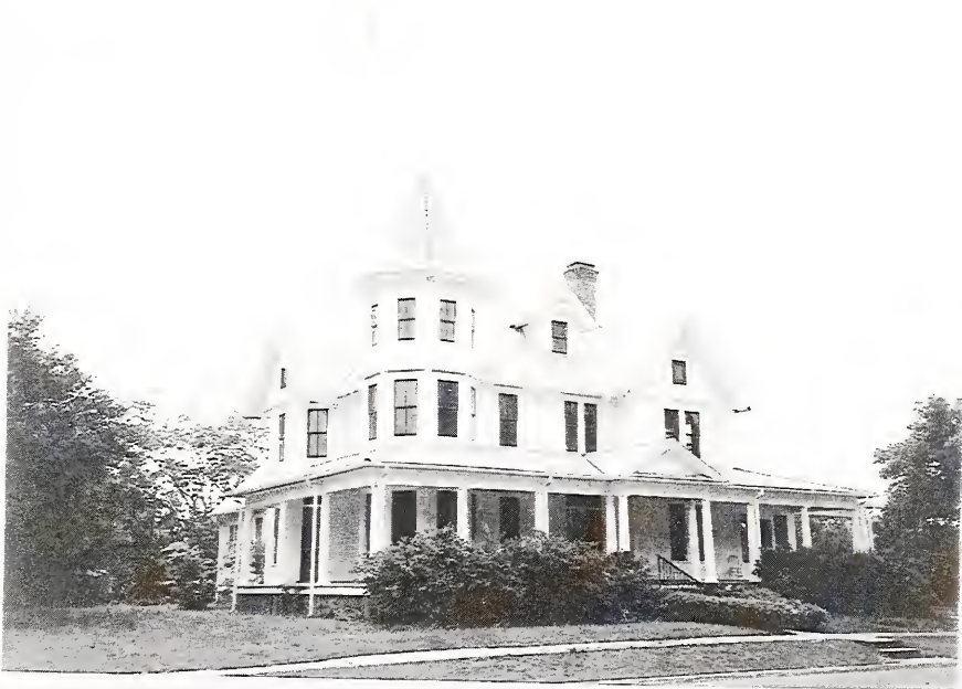
Figure 8. Williams-LeRoy House, 14603 Main Street
