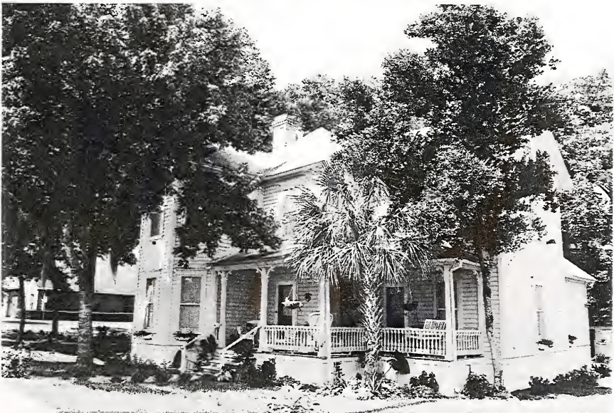
Figure 7. Bell House, 14707 NW 140 Street
