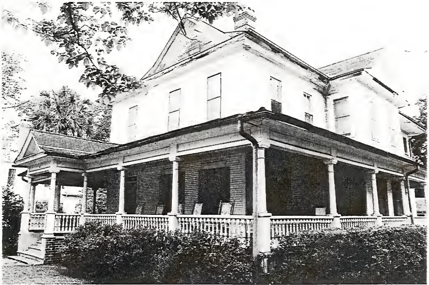
Figure 10. Mizell-Stephens House, 14705 Main Street
