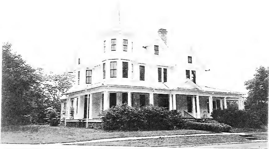
Figure 8. Williams-LeRoy House, 14603 Main Street
