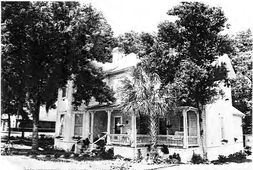
Figure 7. Bell House, 14707 NW 140 Street
