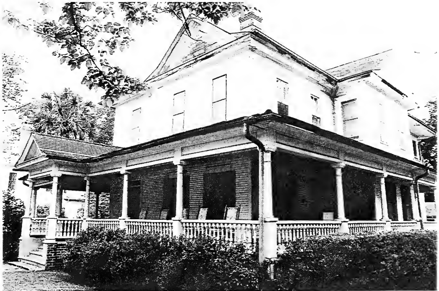
Figure 10. Mizell-Stephens House, 14705 Main Street
