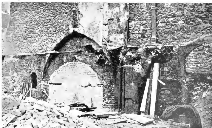
EXTERIOR, NORTH WALL OF NUNS' QUIRE (REMAINS OF SACRISTY)
