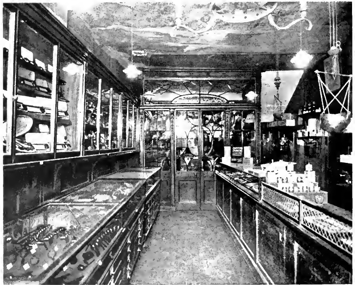
No. 34, HAYMARKET, INTERIOR OF SHOP ( p. 98)
