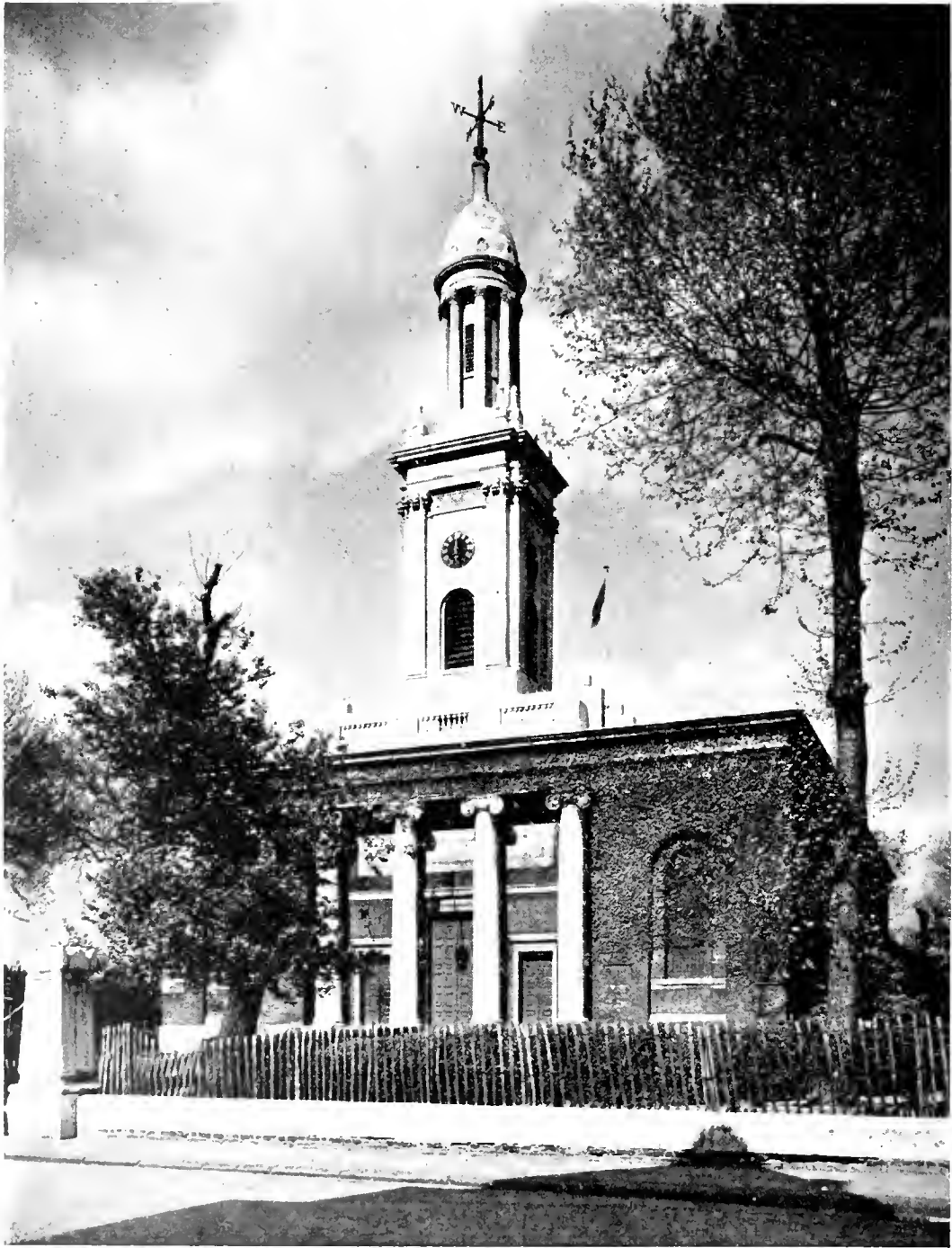
ST. PETER'S CHURCH FROM SOUTH-WEST, 1951 (pp. 95-98)
