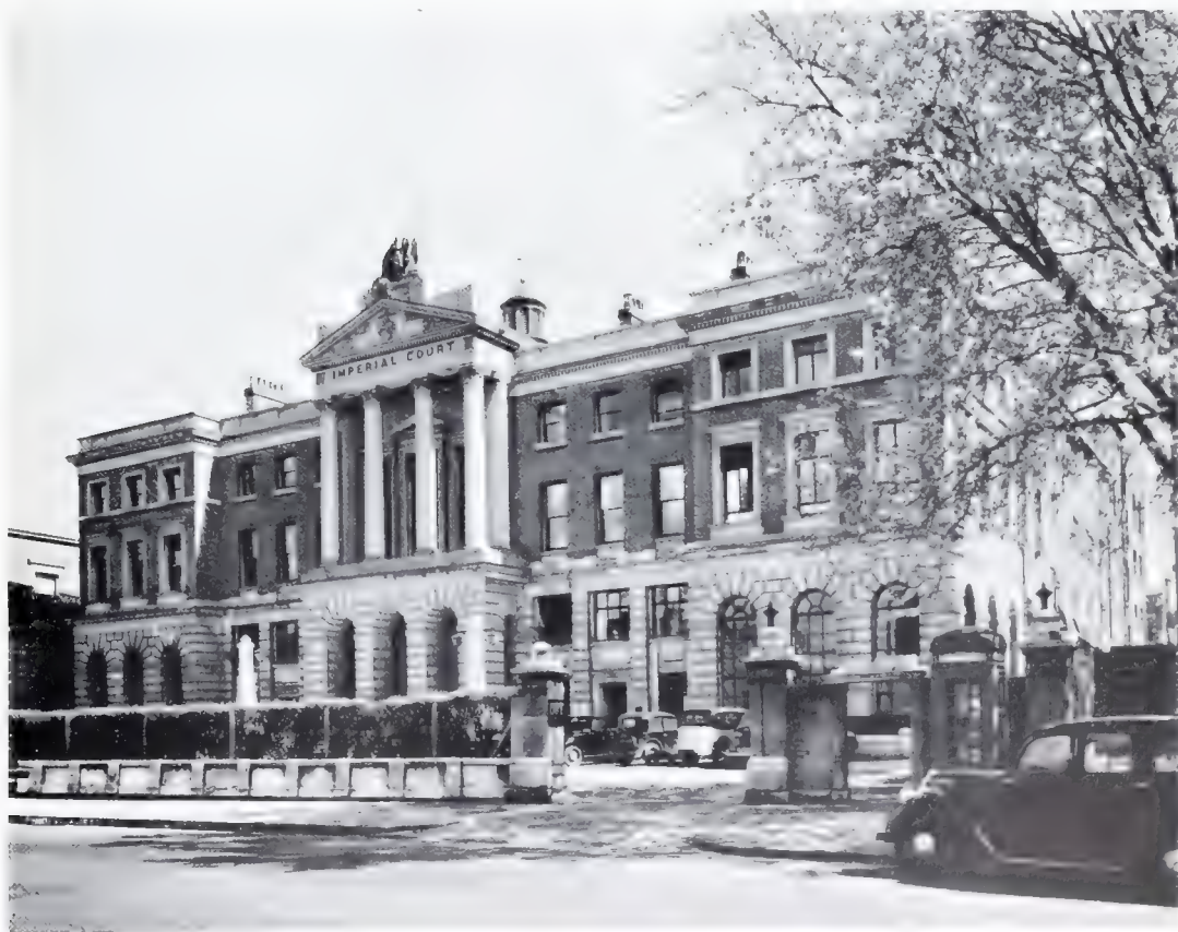
b. IMPERIAL COURT, FORMERLY LICENSED VICTUALLERS' SCHOOL, KENNINGTON LANE, 1836. Henry Rose, architect (p. 43)
