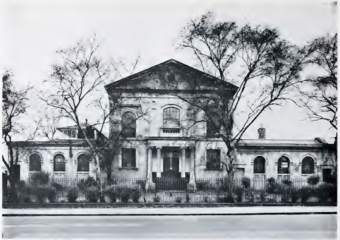
27. CHAPEL ROAD CONGREGATIONAL CHURCH, 1819-21 (p. 179)
