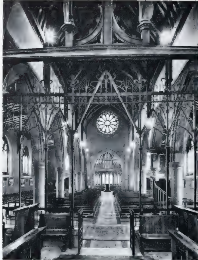
a. Interior, looking west
