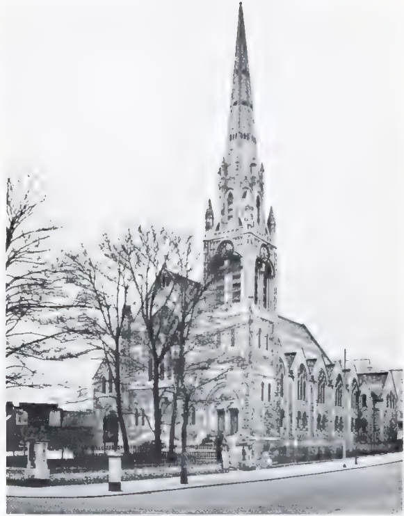
b. ROUPELL PARK METHODIST CHURCH, NORWOOD ROAD, 1879-80. Charles Bell, architect (p. 180)
