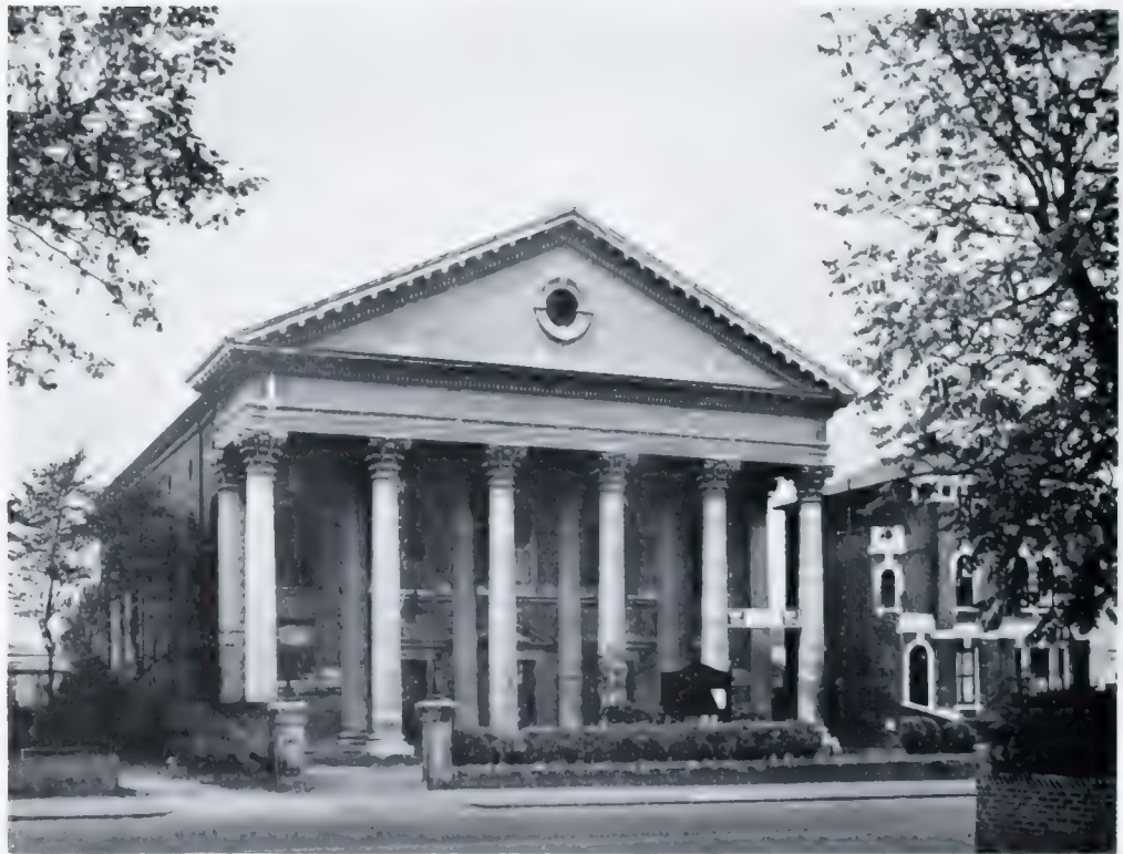
28. TRINITY PRESBYTERIAN CHURCH, Chapel Road, 1862. W. G. Habershon and A. R. Pite, architects (p. 83)
