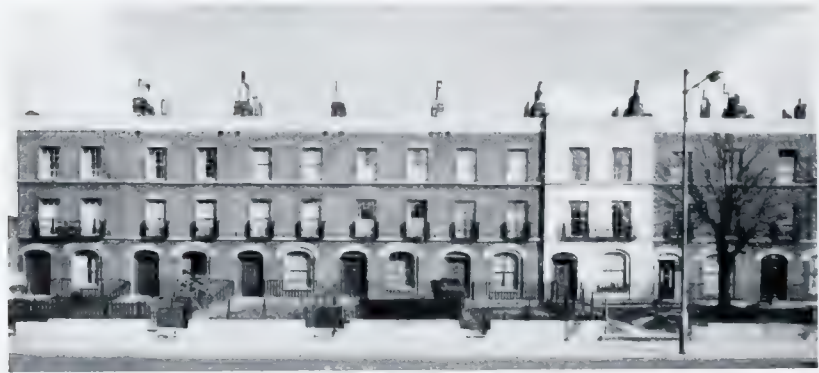
b. Nos. 117-31 BRIXTON ROAD, 1823. Lessee, James Crundall, timber merchant (p. 111)
