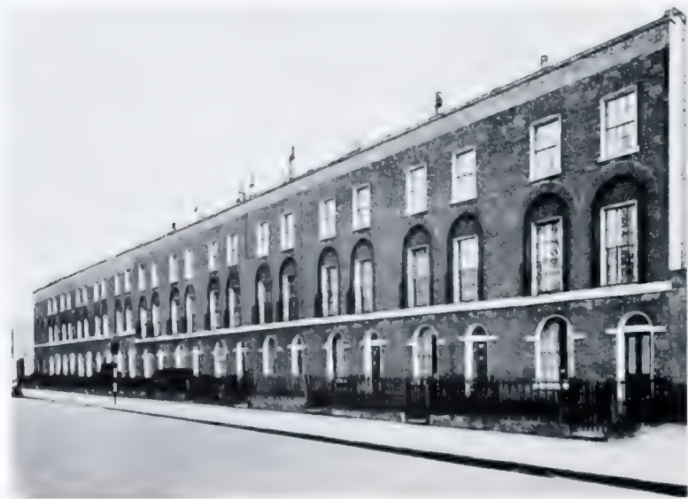
c. Nos. 37-61 HILLYARD STREET, 1822. Lessee, James Crundall, timber merchant (p. 111)
