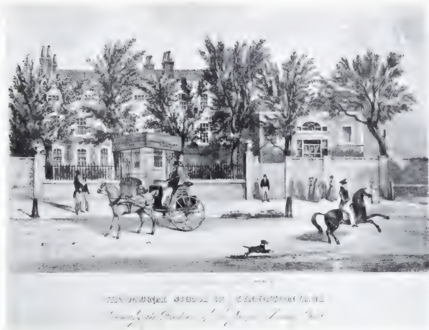
a. LICENSED VICTUALLERS' SCHOOL, KENNINGTON LANE, demolished c. 1836 (p. 43)
