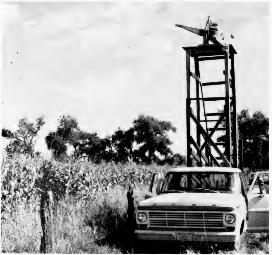
Fig. 4 Gas-powered blower on dispersal tower.
