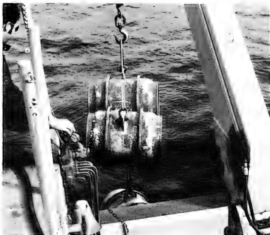
Figure 2. Lowering steel drums from which sample line will be suspended in the ocean.
