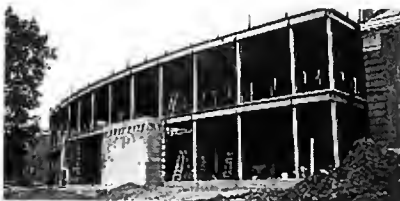
Construction continues on the Clyde P. Jacobs Fitness Center.
