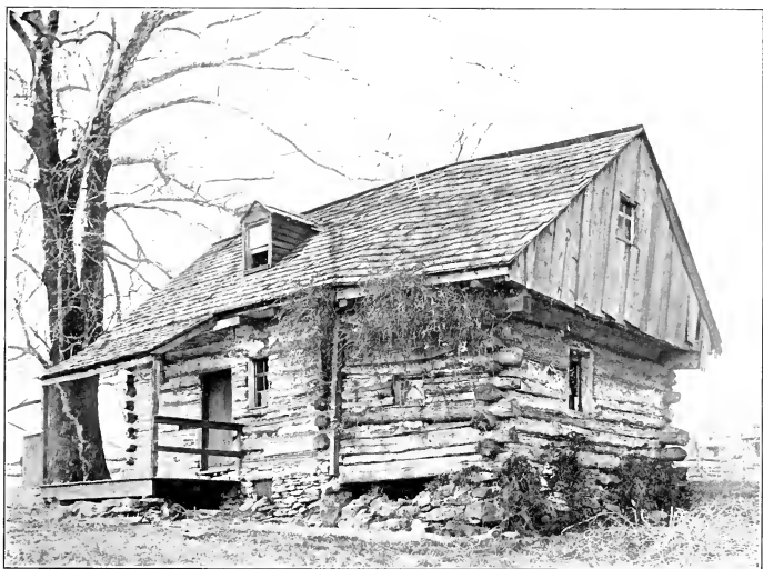
"Swedish log cabin" situated "on the west bank of Darby creek about a quarter of a mile above Clifton." The above (built in the 18th century) shows many characteristics to be found in the log cabins erected by the Swedes and Finns in their native country; the extension of the second story, "the porch-roof," etc.
