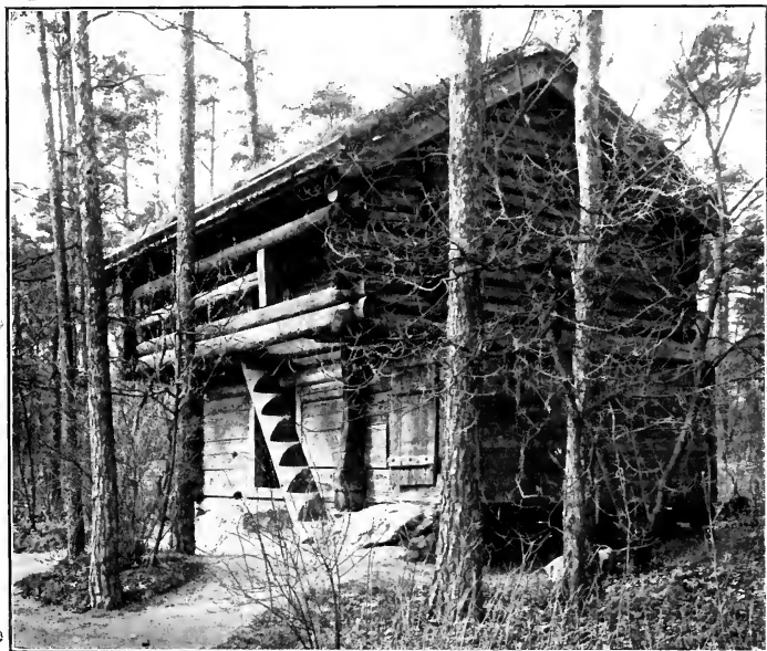
Storehouse, (now at Skansen, Stockholm), showing the extended "balcony" and the "log-ladder" leading up to it.
