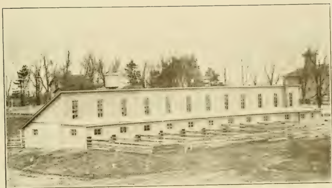
Illinois Experiment Station Hog House—Exterior
