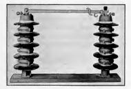
Fig. 12.—Disconnecting switch with built up insulator column.
