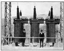
Fig. 79.—General Electric Co. oil circuit breaker type KO36.
