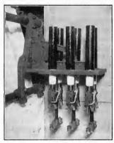
Fig. 81.—Westinghouse oil circuit breaker, type F-1.
