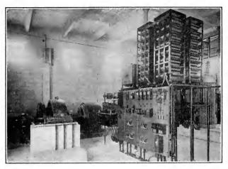
Fig. 208.—General Electric Co. automatic substation with M.G. set.
