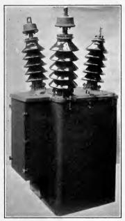
Fig. 131.-Westinghouse outdoor metering equipment.
