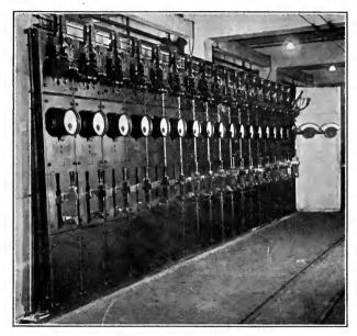
Fig. 180.—Westinghouse three section railway switchboard.
