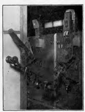
Fig. 48.—Westinghouse carbon circuit breaker, type CA.
