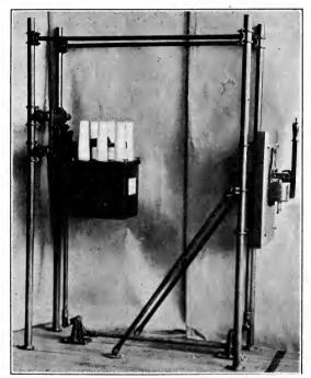
Fig. 57.—Condit Electric & Mfg. Co. oil circuit breaker, type E4, hand operated, remote control.
