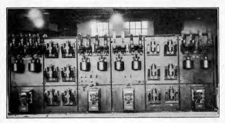
Fig. 214.—Field & exciter switchboard for Inawashiro.
