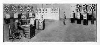
Fig. 228.—Control pedestals & posts of Ontario Power Co.
