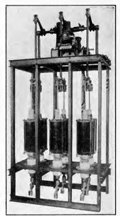
Fig. 74.—General Electric Co. oil circuit breaker type H6 with parallel pots.
