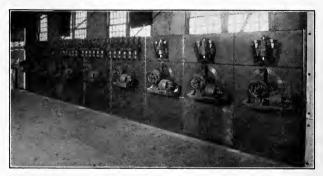
Fig. 213.—Field & exciter switchboard for Rio de Janeiro.
