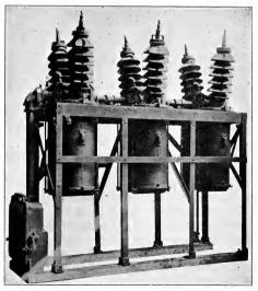
Fig. 95.—Westinghouse type "G-11" outdoor oil circuit breaker, 400 amps., 73 K.V.
