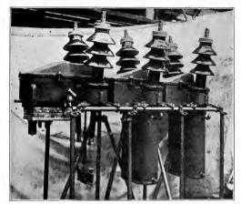
Fig. 94.—Westinghouse type "G-11" outdoor oil circuit breaker, 400 amps. 37 K.V.
