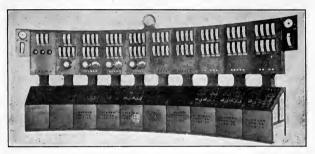
Fig. 232.—Control desk with vertical edgewise meters.
