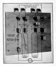
Fig. 200,-Cutter circuit breaker for three-wire generator.
