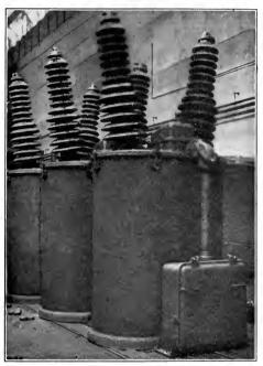
Fig. 98.—Westinghouse type "GA" outdoor oil circuit breaker, 400 amps., 135 K.V.
