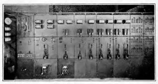
Fig. 222.—Panel switchboard, hand operated breakers—General Electric Co.
