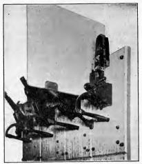
Fig. 51.—Westinghouse remote-control 1500-volt breaker.
