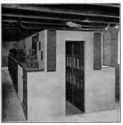
Fig. 87.—Westinghouse type "C" circuit breaker installation.
