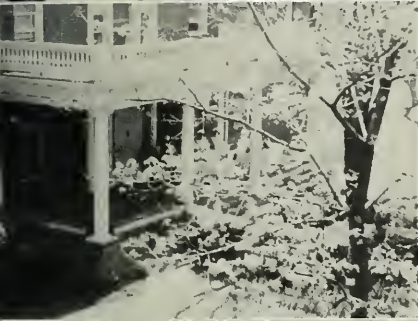
North Center Hospital's nurses residence.
