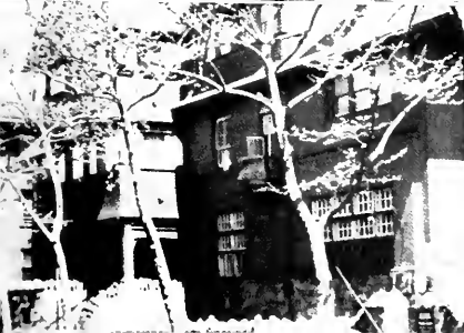
Looking north on 20th Street.
