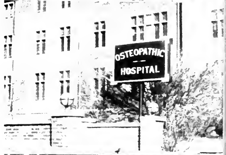
O.H.P.'s main entrance on 48th Street.
