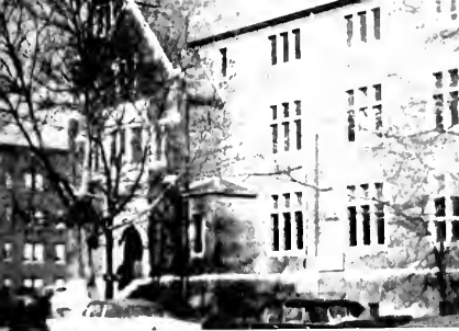
The College entrance on 48th Street.
