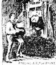
FORGING A PLOW-POINT
