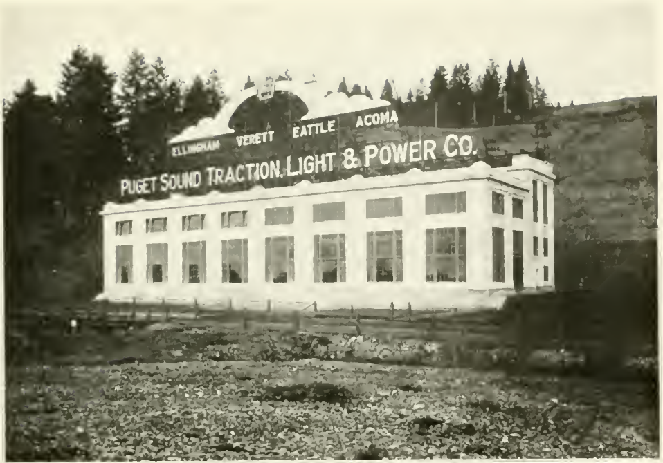
WHITE RIVER POWER PLANT, LOCATED BETWEEN SEATTLE AND TACOMA
