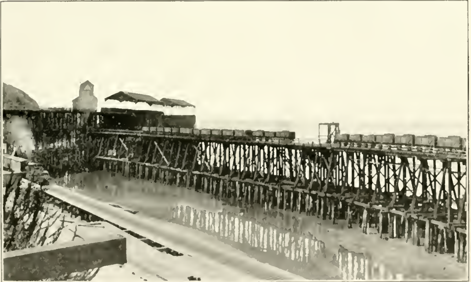
OLD COAL BUNKERS WHICH STOOD FOR MANY YEARS JUST BELOW THE STADIUM
