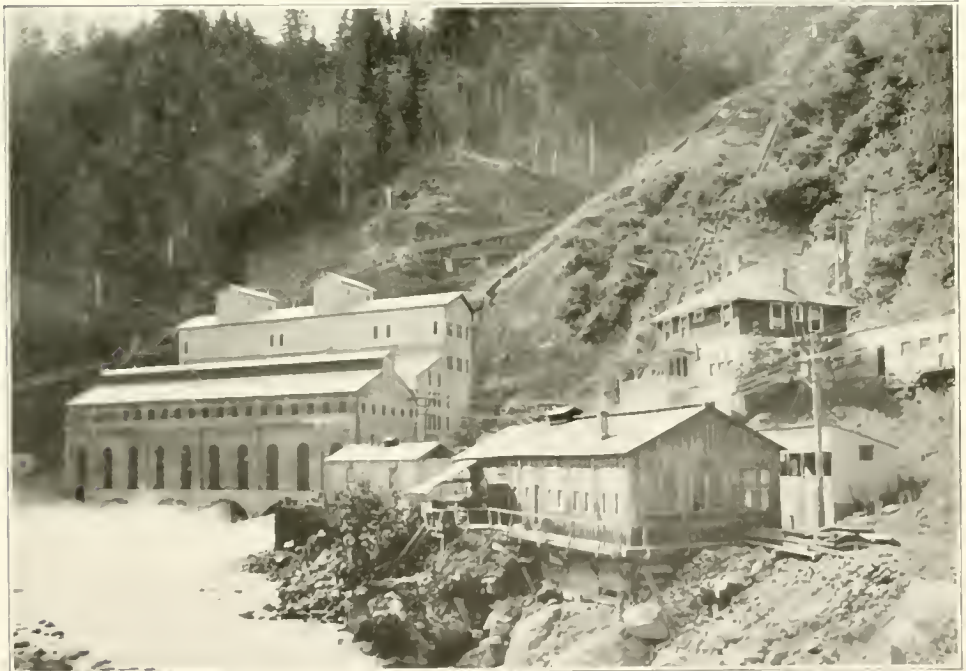
ELECTRON PLANT ON THE PUYALLUP RIVER Great power development by the Stone & Webster Engineering Corporation
