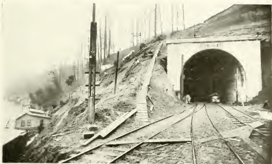
WEST PORTAL OF THE NELSON BENNETT TUNNEL
