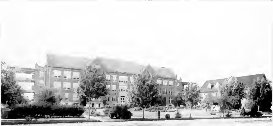
NORTHERN PACIFIC HOSPITAL Built in 1905 at a cost of $175,000
