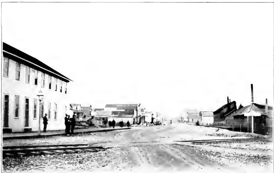
LOOKING NORTH ON PACIFIC AVENUE FROM SEVENTEENTH STREET, IN 1883
