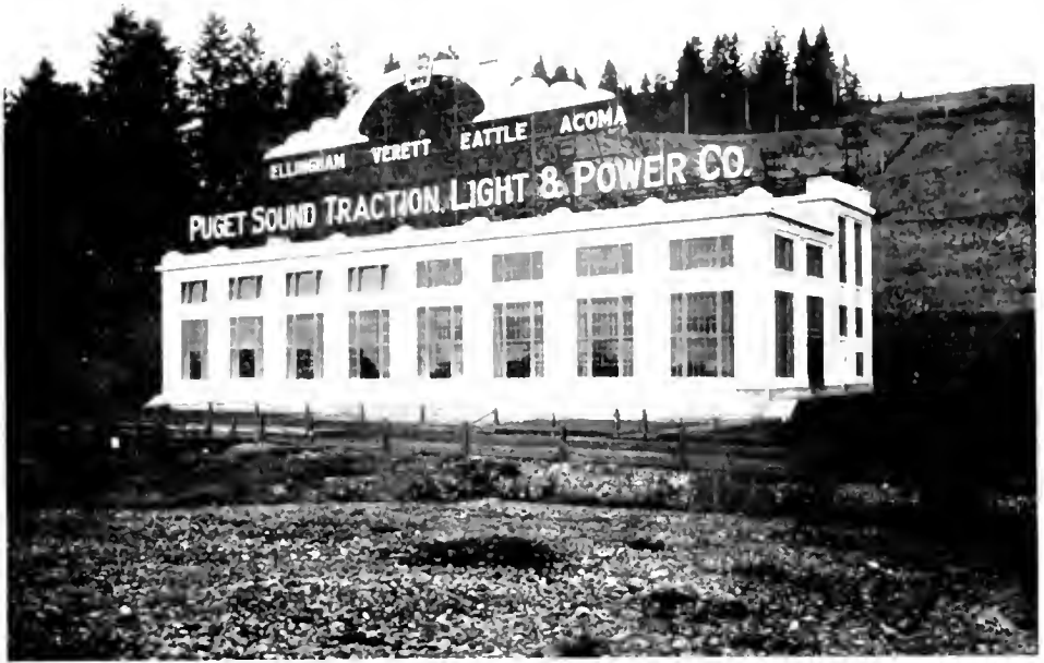
WHITE RIVER POWER PLANT, LOCATED BETWEEN SEATTLE AND TACOMA
