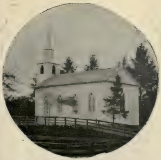
ST. PETER'S, TYRCONNEL. Erected in 1828.
