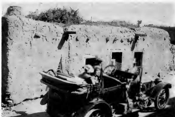
In front of "the oldest house" in the United States, located on a narrow street in Santa Fe, New Mexico, and said to date from 1530. It is of adobe construction—mud and straw—and was formerly two stories in height. A Mexican family makes it its home
