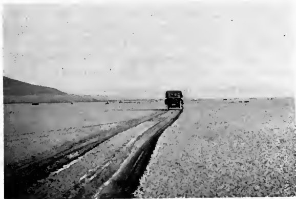
On the Lincoln Highway across Nevada there are several of these mud flats. When dry they afford excellent going, but when wet become absolutely impassable for motor traffic and have caused great hardships and delay to transcontinental motor tourists. Extensive improvements, now under way, will make for comfortable travel through this region
