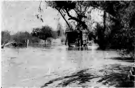
The crossing of Indian Slough on the Colorado River, near Blythe, California, with the first transcontinental truck, closely resembled submarine work
