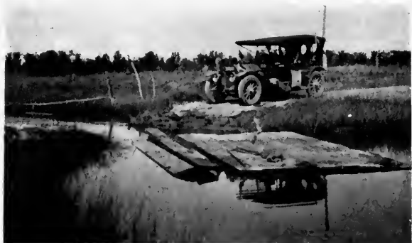
This situation, encountered in Montana, necessitated the taking apart and reconstructing the bridge. Laborious and slow but counted as all in the day's work
