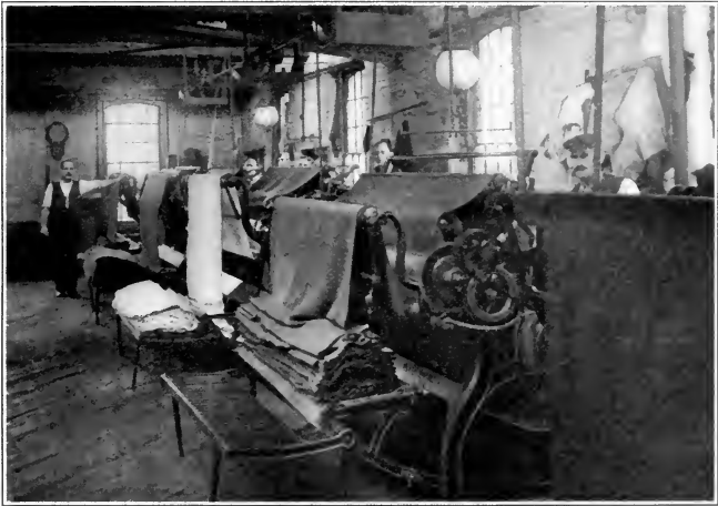
SHEARING AND SINGEING MACHINES
