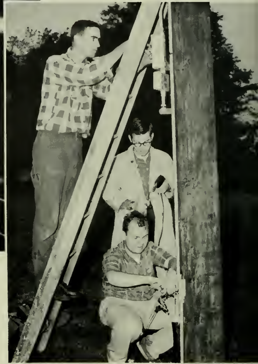
The "fix-it" crew on the job
