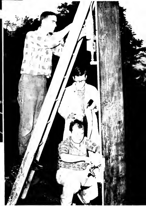
The "fix-it" crew on the job
