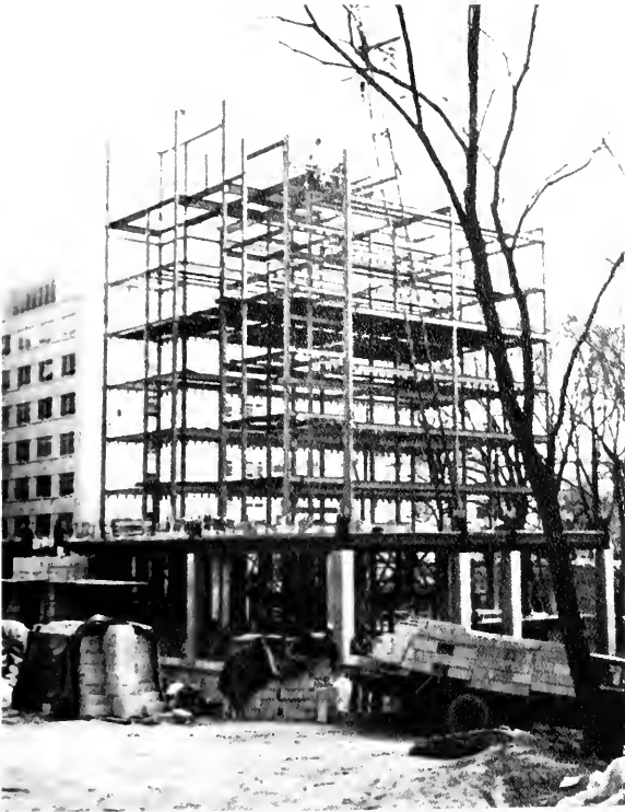
Construction proceeds on the addition to Hughes Hall.
