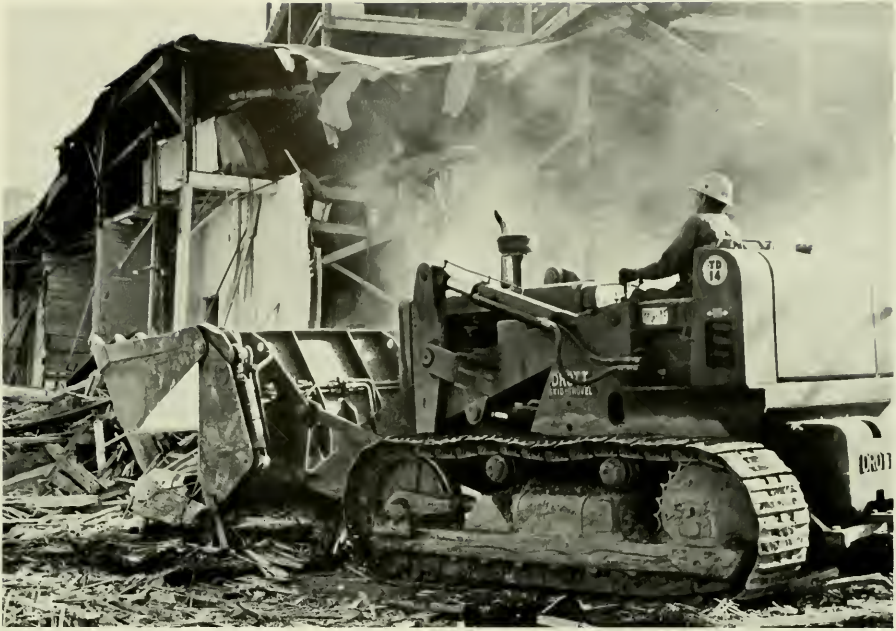
A bulldozer makes way for a new dormitory by removing the vacated "old" McCabe Building.
