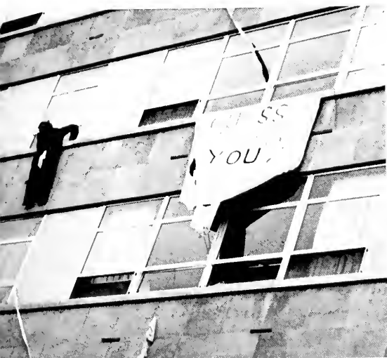
McDowell advertises that all electricity was off.
