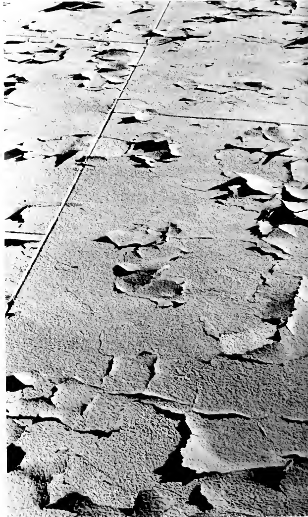
Peeling Paint on the walls of Mary Graydon Center. John Purdy
