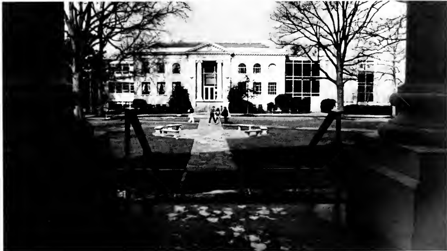
A view of Battelle from Hurst Hall/John Quale
