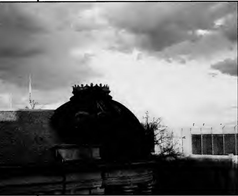
McKimley Building/John DeLuca
