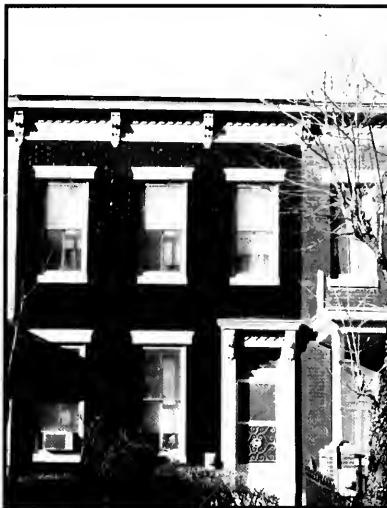
left: What is this house's fate? above: Renovation...
