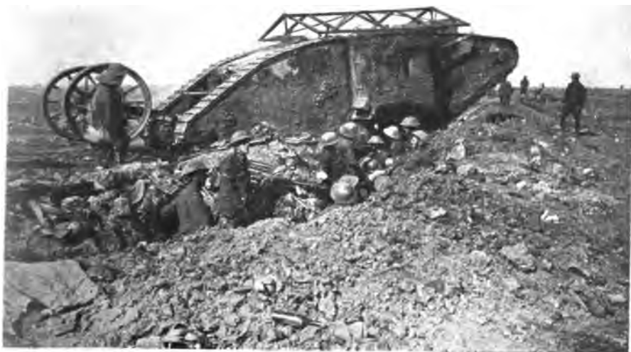
THE ORIGINAL THIEPVAL MARK I. TANK WITH ANTI-BOMB ROOF AND "TAIL"
