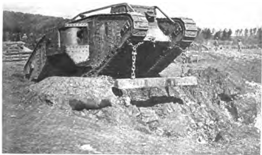
THE UNDITCHING BEAM IN ACTION
