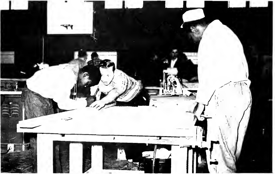
Carpentry in action.
