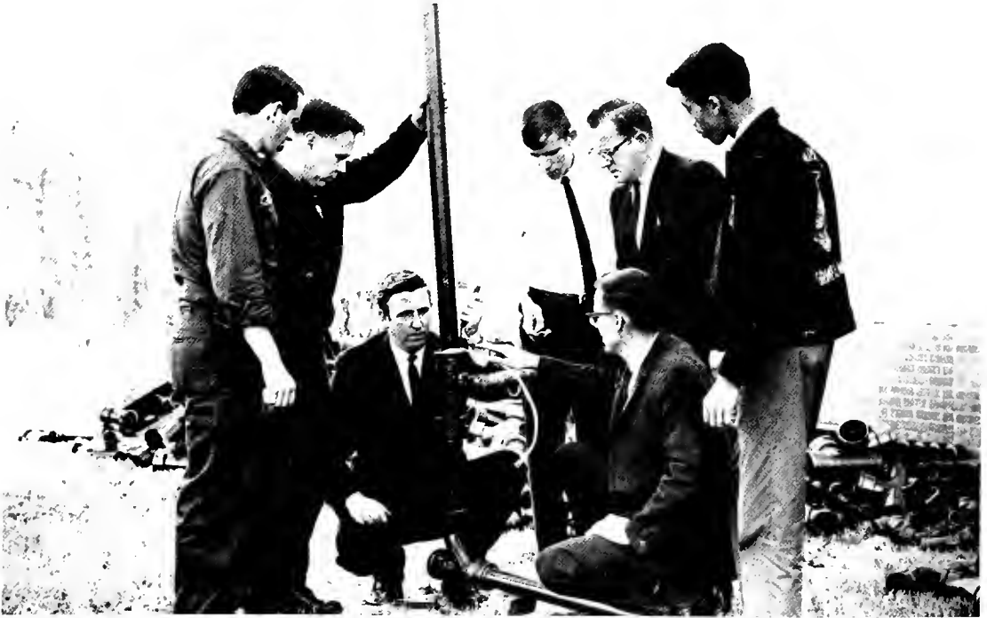
"We start from the ground up."
