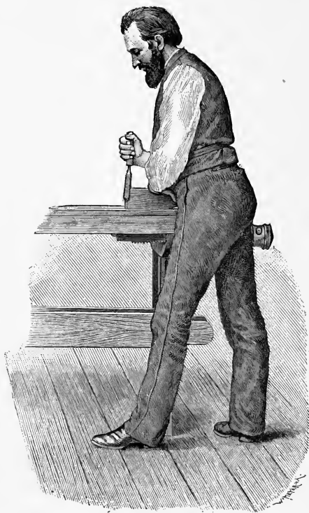
Plate VI. Position : Perpendicular chiselling.
